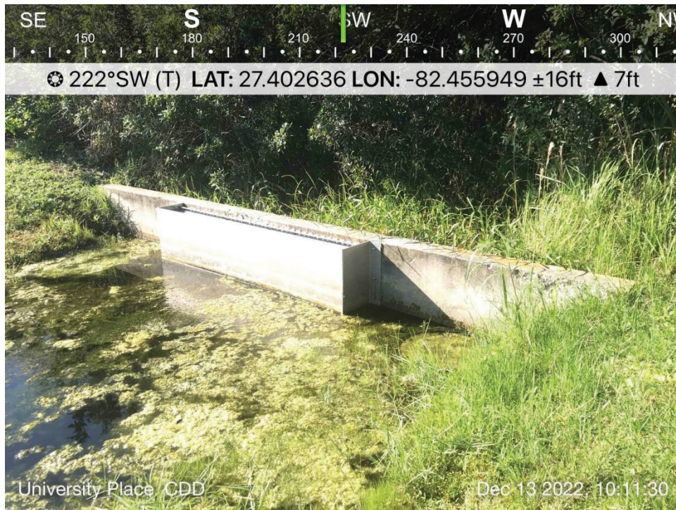
POND 2 – View of CS #UP2 Operating normally, low water levels, recommend removing PVC grate from weir.
