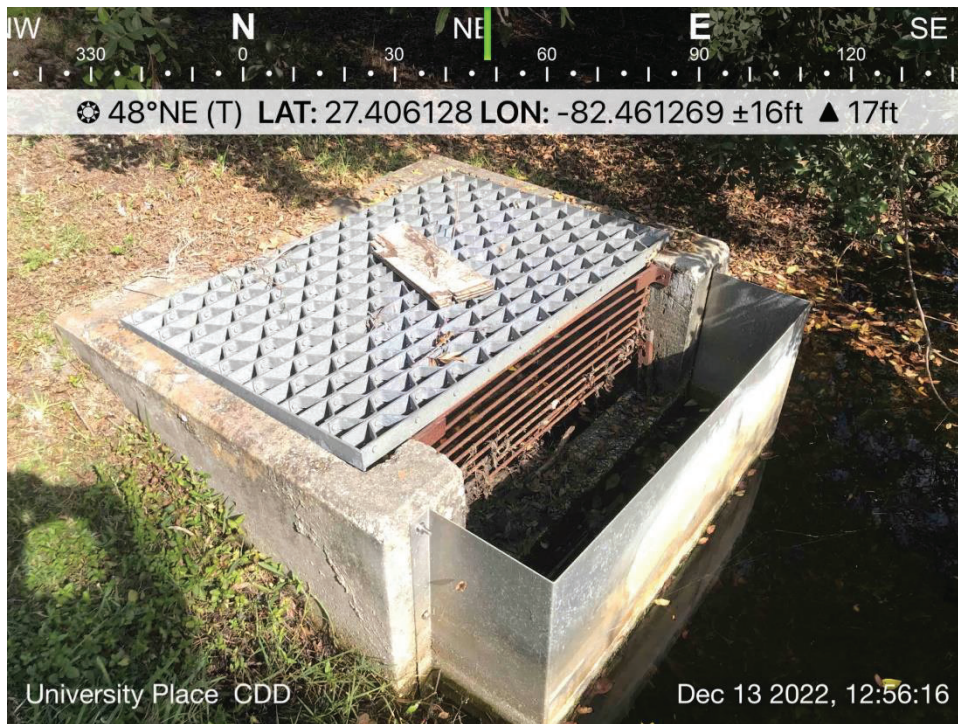
POND 10 – View of CS #UP10. Operating normally, low water levels, recommend removing metal grate at weir.
